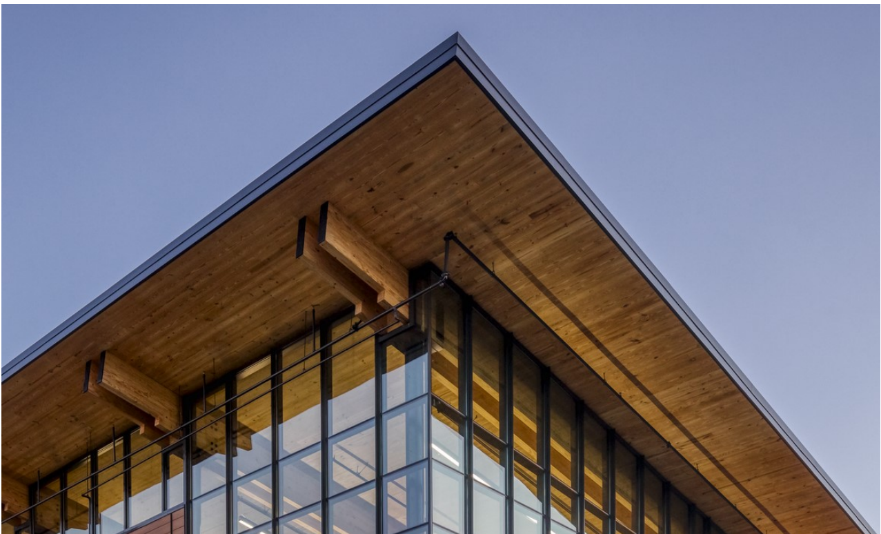
Panels cantilever in two directions at the Andy Quattlebaum Outdoor Education Center in Seneca, SC / Cooper Carry / Photo Jonathan Hillyer
